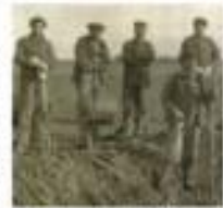
Men from the drainage crew using hand tools.
